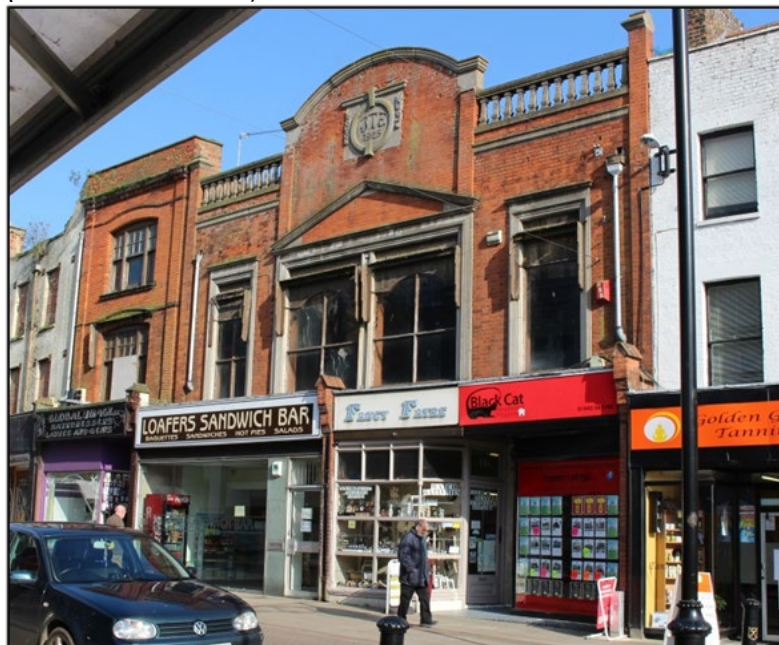
13-17 High Street – grant application approved for new shopfronts, first floor conversion and brickwork repair
